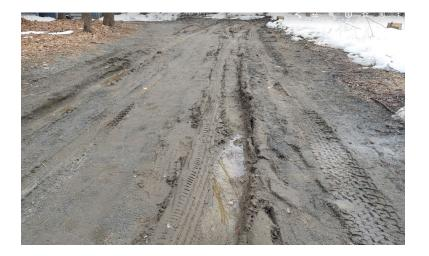
In front of the (4) dumpsters, the road surface is scraped through to clay, and also needs grading and resurfacing.
